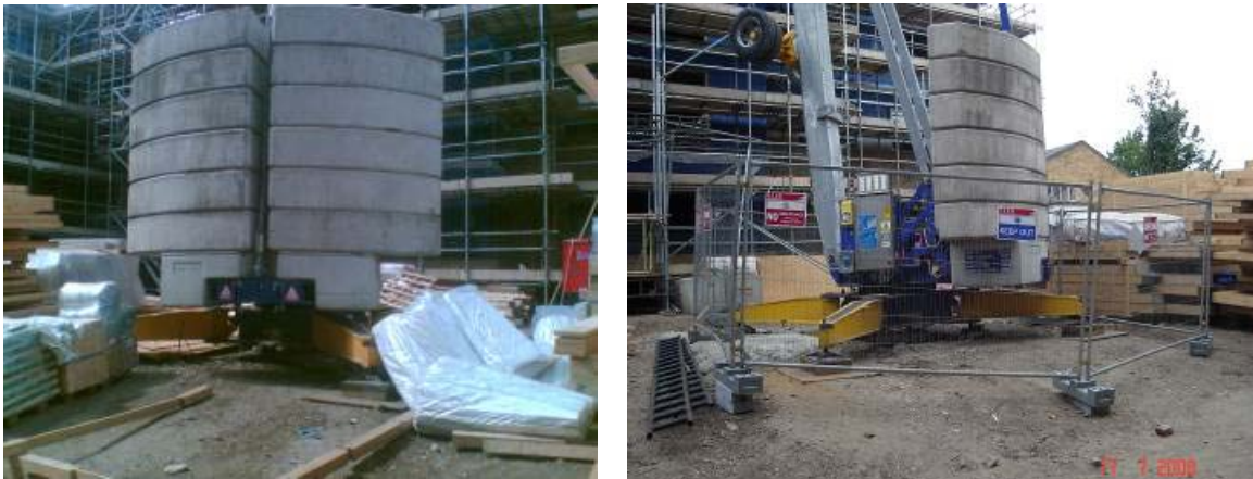
Figure 6 - Unprotected and Protected Base of a SETC
