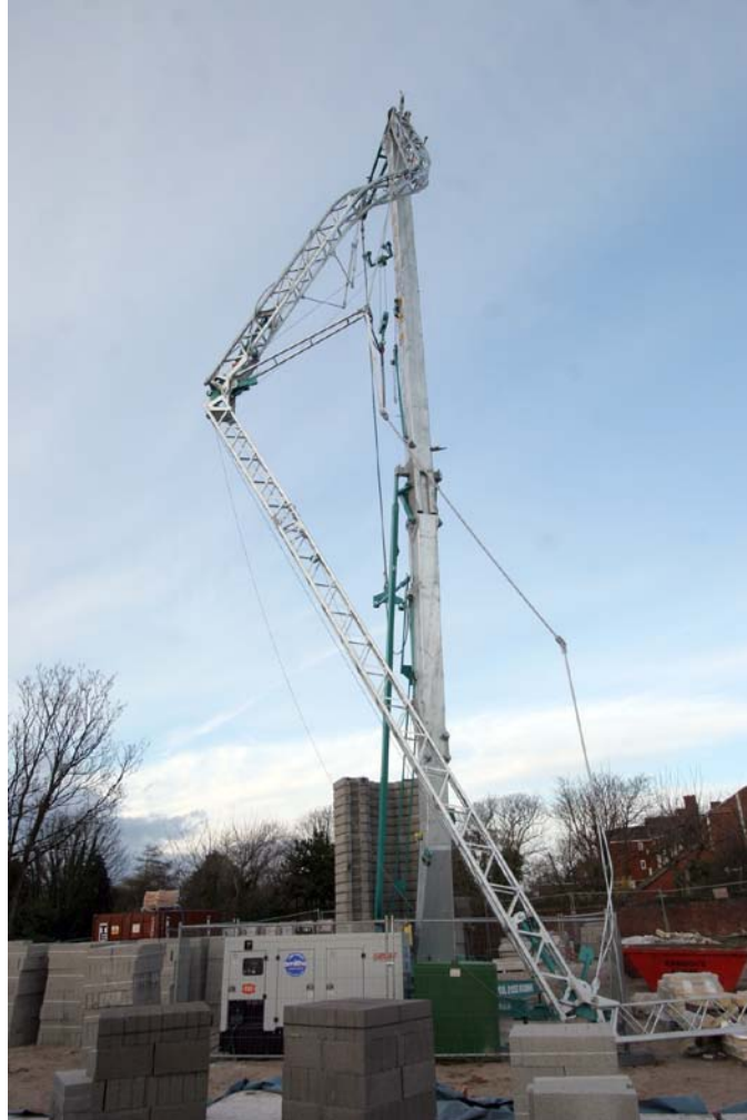
Figure 9 - Result of Folding the Jib in High Winds
