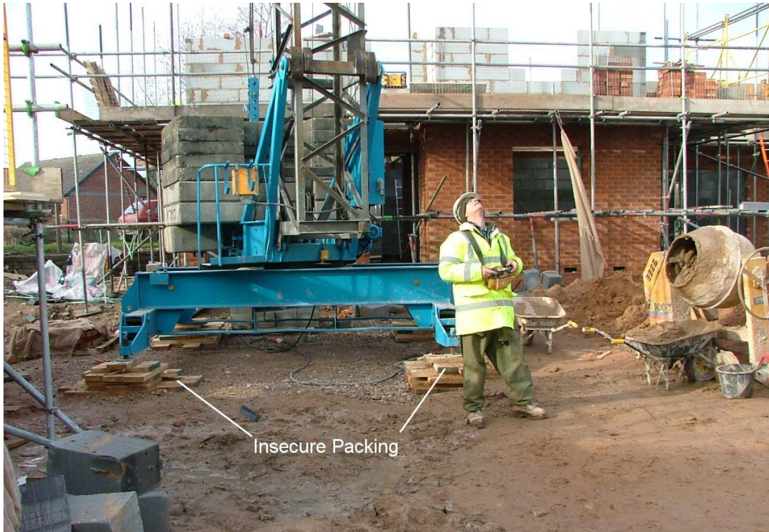
Insecure Packing Under Outriggers (See 5.3)
