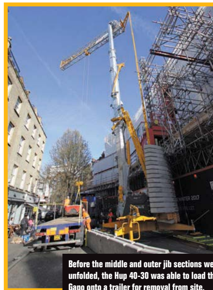
One of the 15 counterweight blocks being installed using the Hup's integral ballasting derrick.
